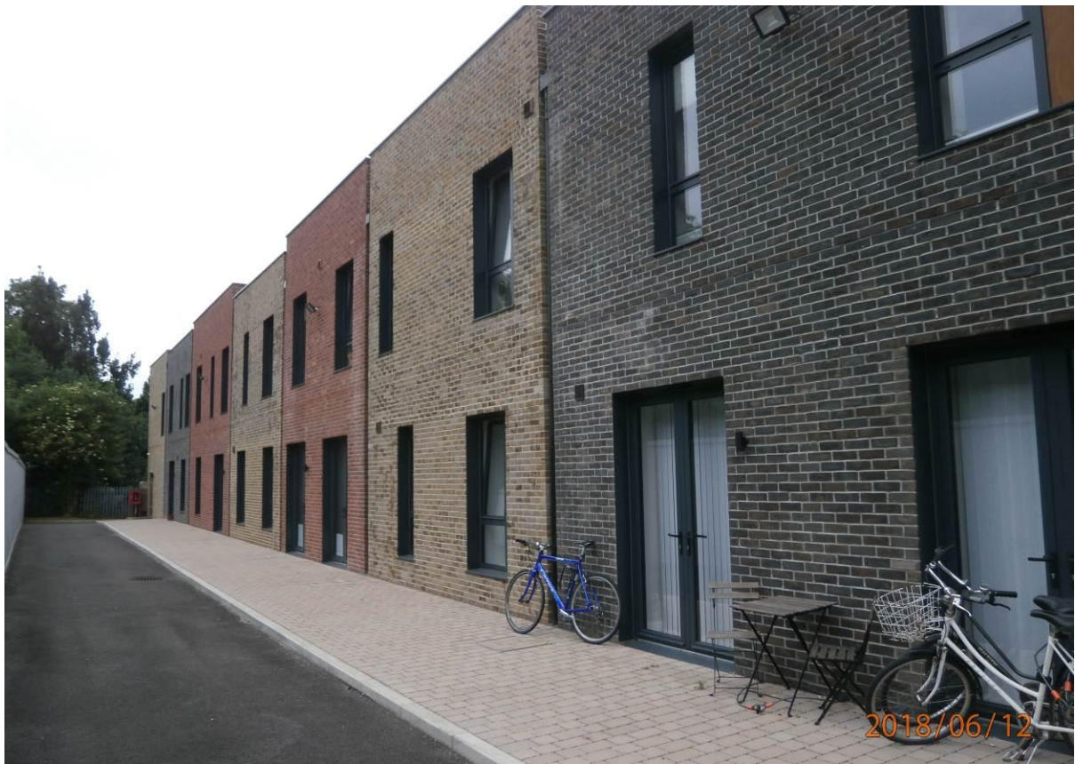
West elevation of Cotton Exchange (former factory building):
